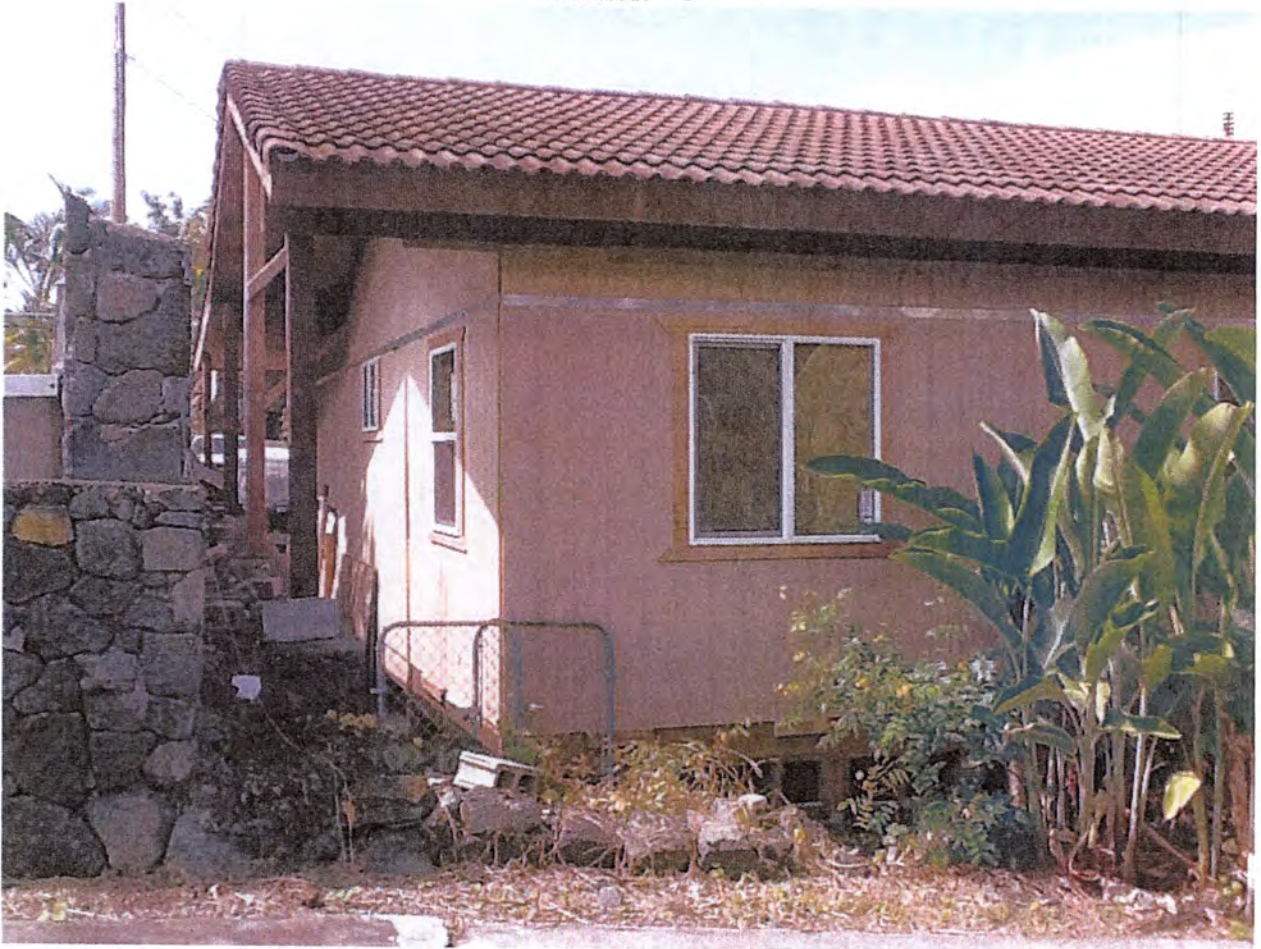
Depicts the unpermitted structure. Note that there is a metal stake denoting the property line to the right side of the rock wall.
