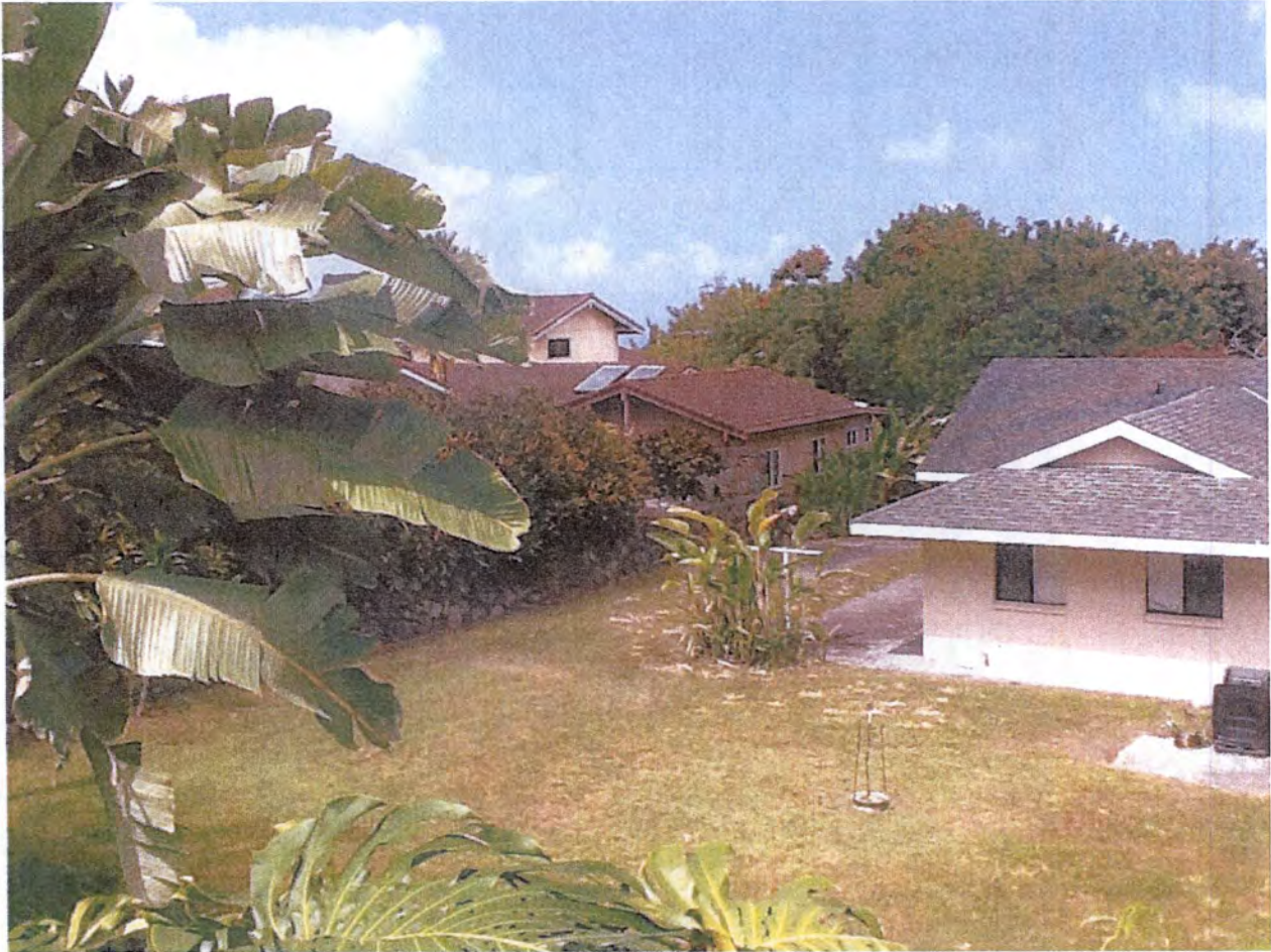
Depicts the structure as seen from the right-of-way from Kiwi Street. It is the structure with the brown roof behind the foliage, immediately in front of the roof with the two solar panels.
