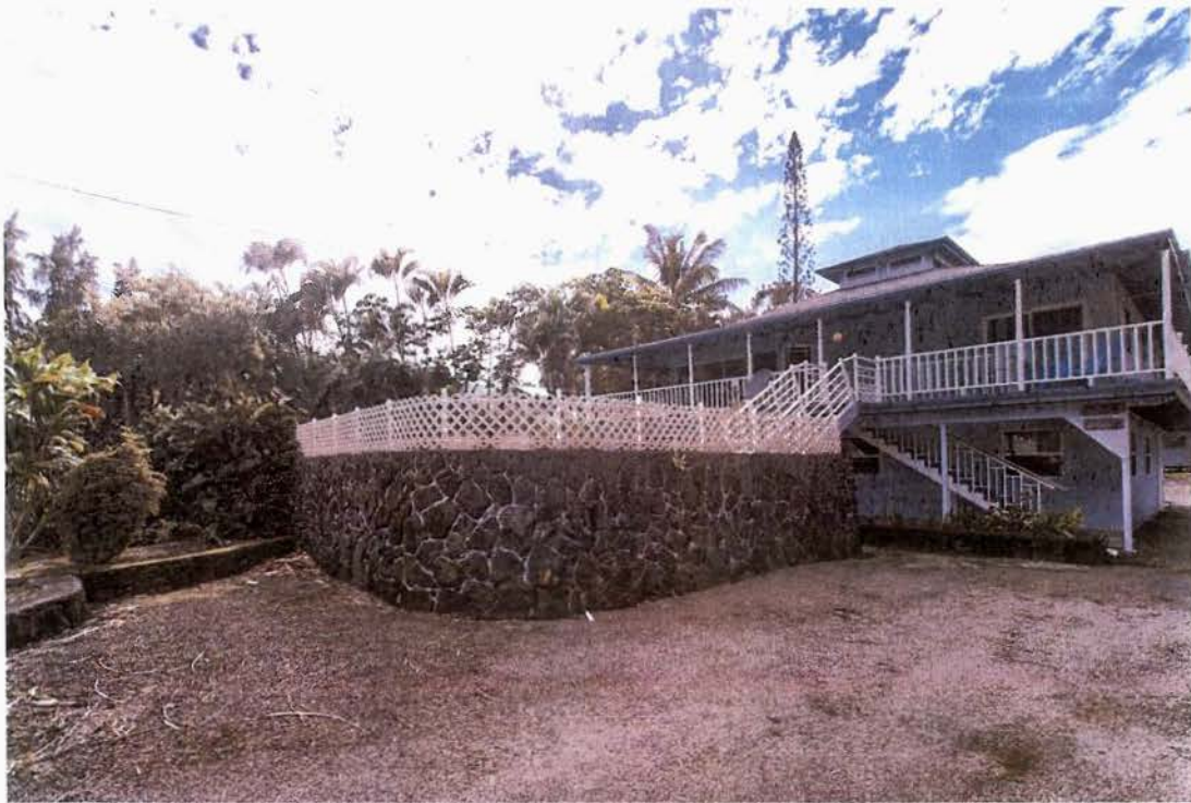
Figure 3b. View to southwest of Rock Wall surrounding pool and deck.
