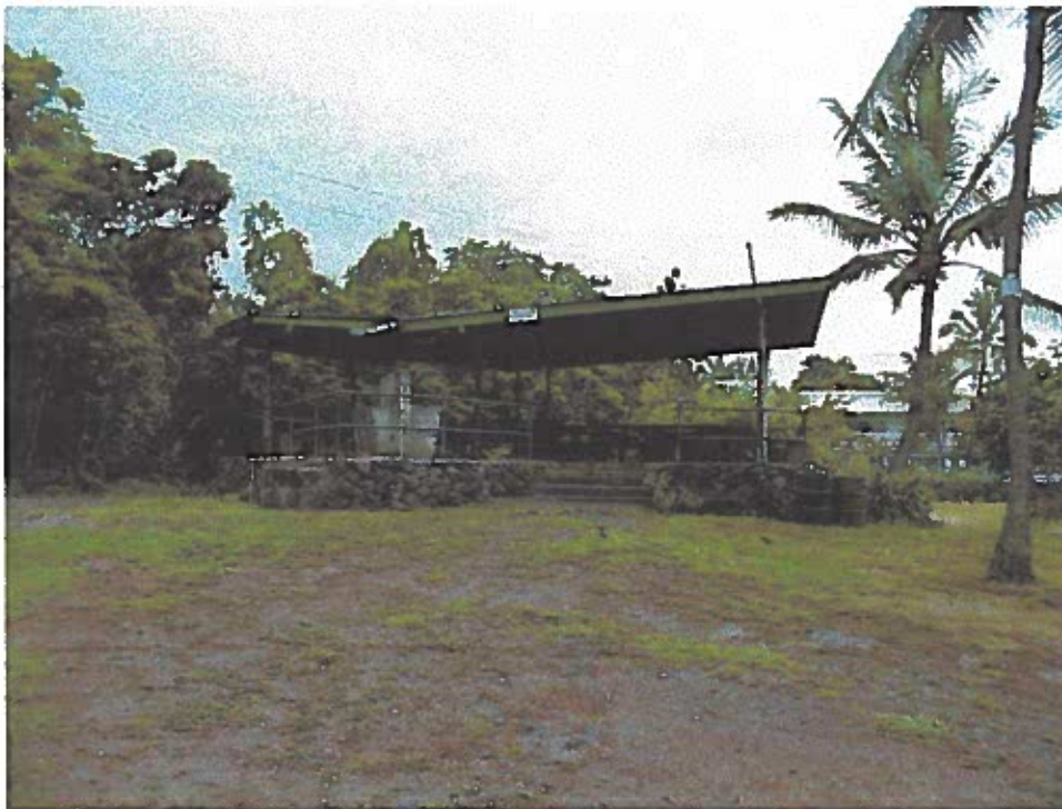
Existing pavilion to be replaced by pavilion/restroom facility.
