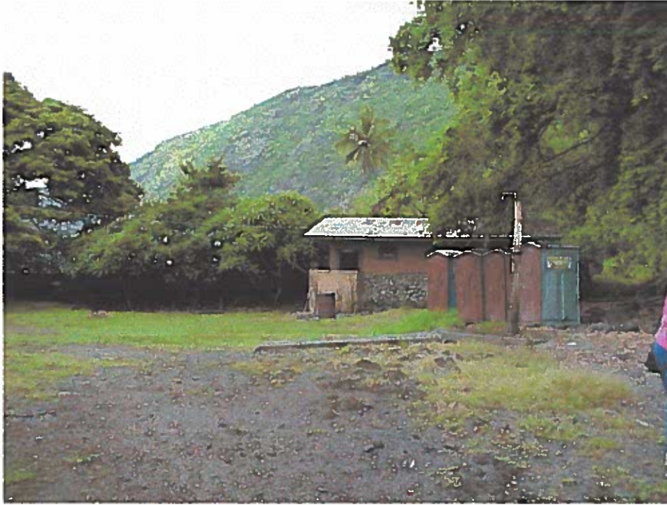
Demolish existing restroom/tool shed; replace shower.
