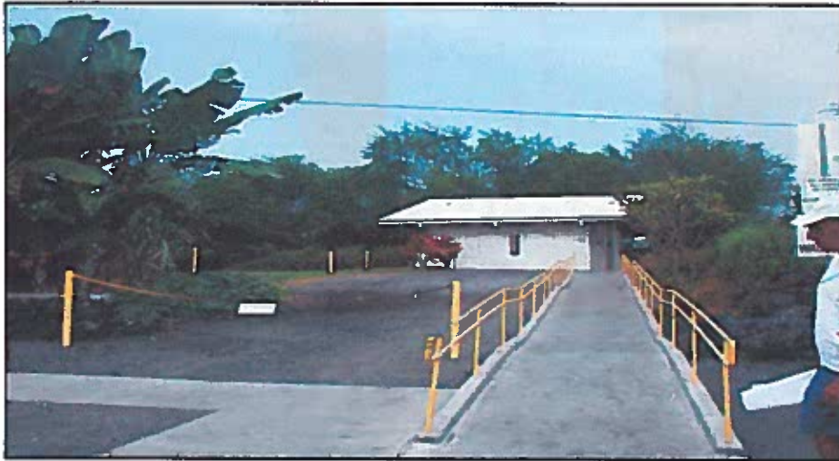
Figure 15. View mauka, Ho'okena Beach Park restrooms. The pro- posed Pavilion would be constructed to the right, behind the rock wall where the banana and sugarcane cur- rently stand.
